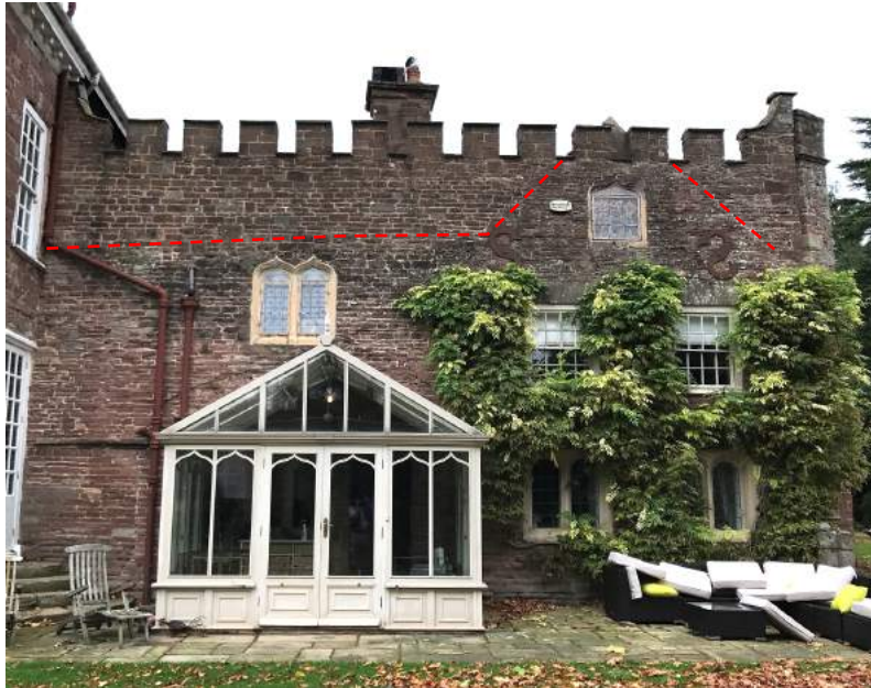
Figure 10 South elevation, changes in patina of masonry indicated by dotted red line.
