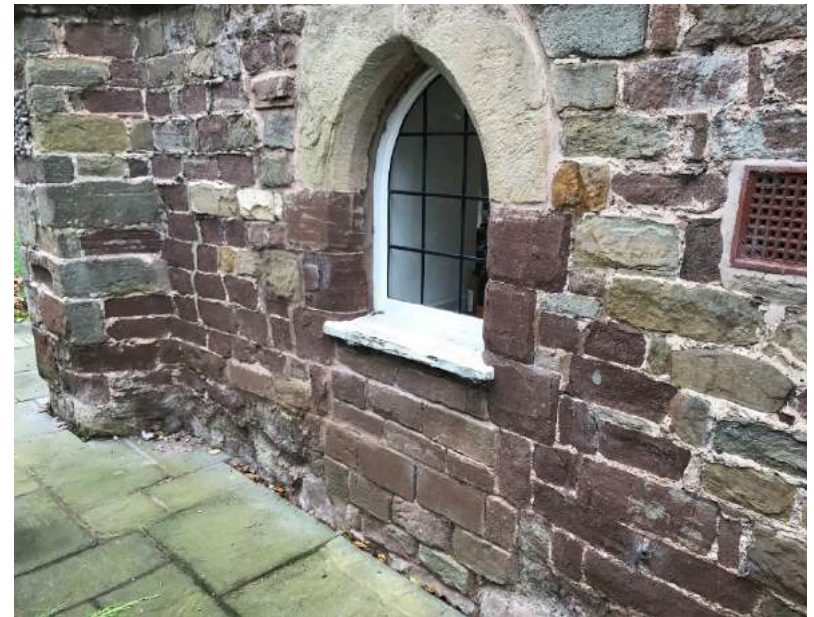
Figure 17 Former door in the north elevation.
