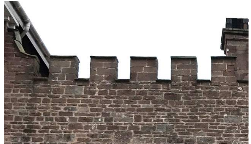
Figure 23 Detail of crenulation on south elevation.
