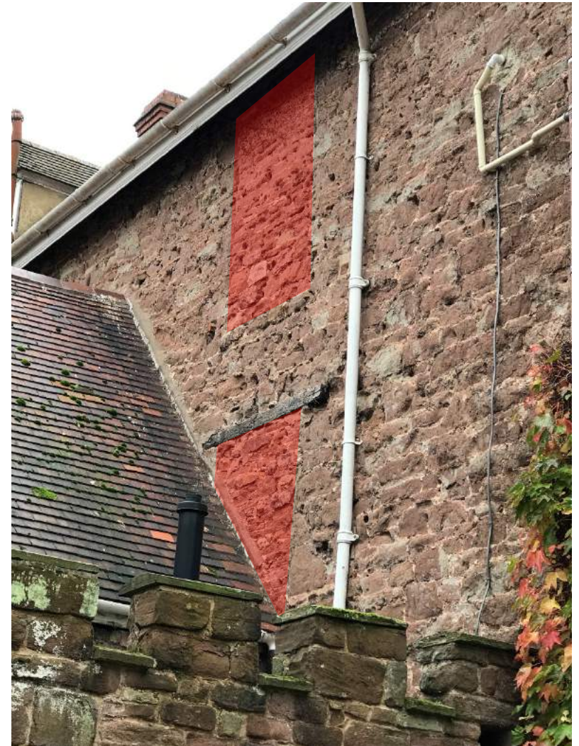
Figure 27 Western range, east elevation; blocked stair windows highlighted red.
