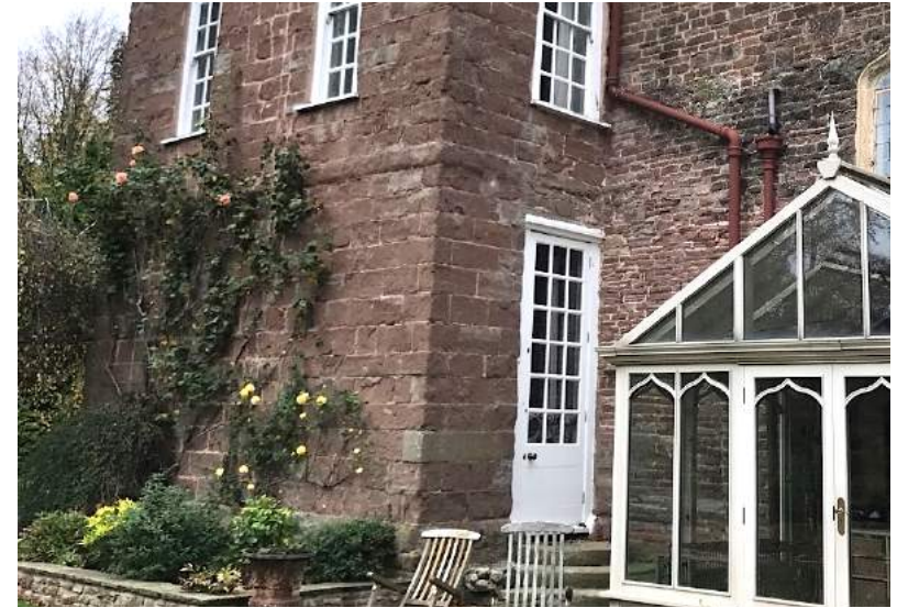
Figure 12 South elevation; detail of junction between deflected wall & fenestration of western range.
