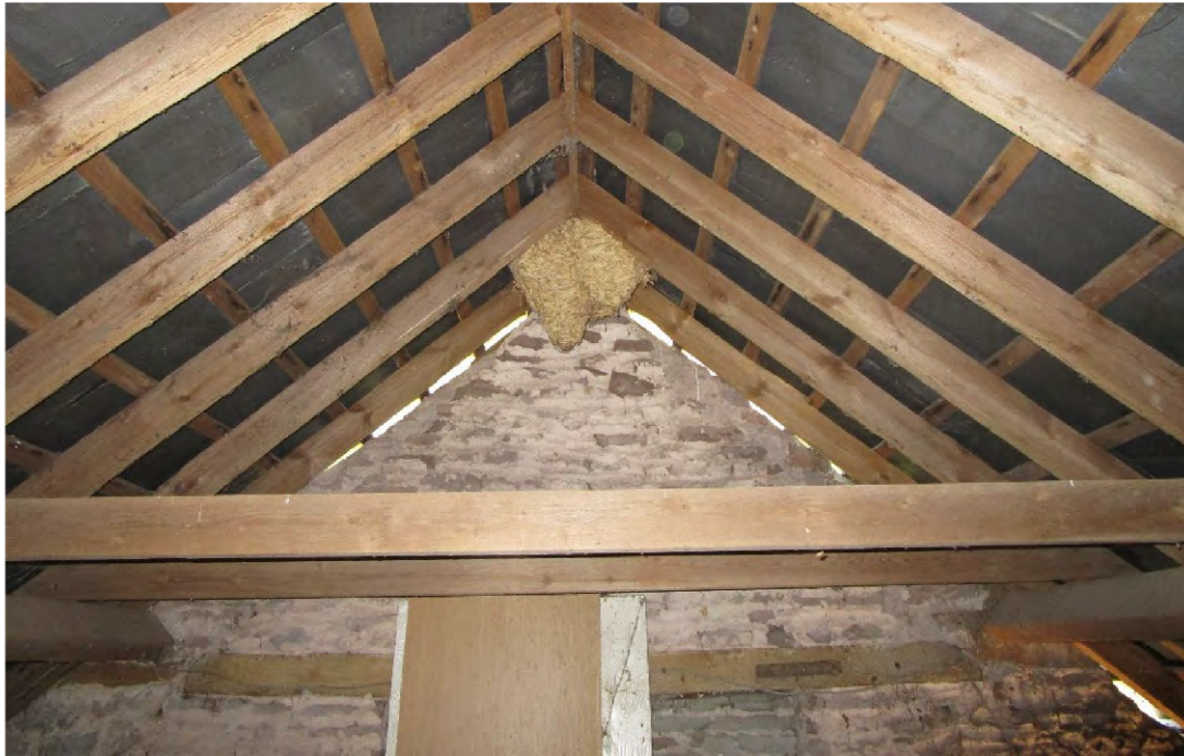
Figure 8: Northern gable end with direct access gaps and wasp's nest
