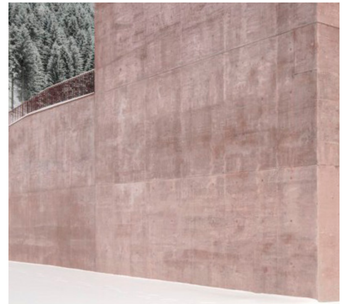
Red pigmented concrete (for the exposed concrete floor)
