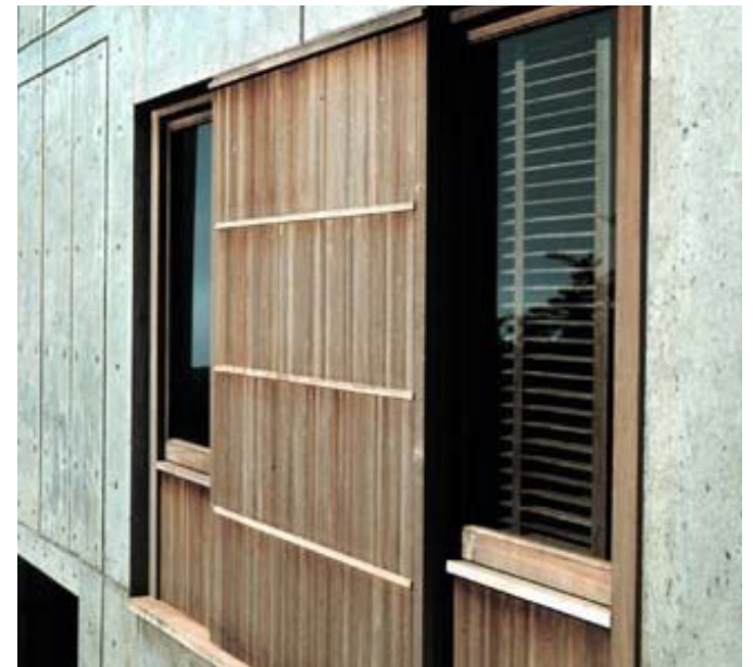
Timber windows 'inserted' into opening
