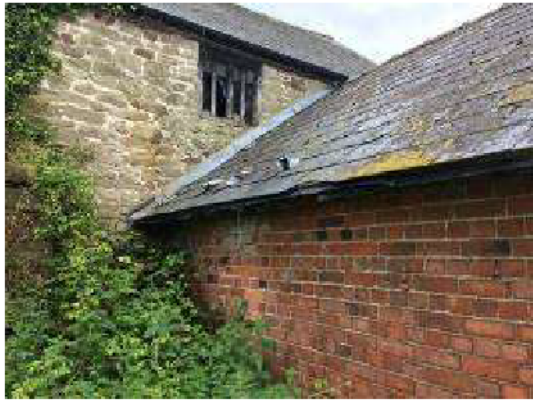
Plate 21: Barn 2 – lead ventilation previously installed bat access points?
