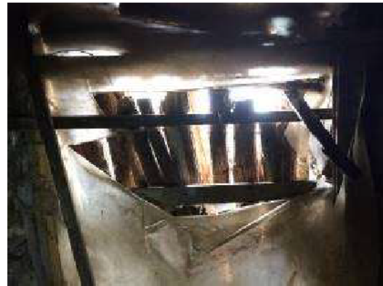
Plate 28: Granary – partially blocked unglazed window at ground-floor level in west gable.
