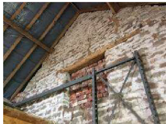
Plates 15 and 16: Barn 1 – Central room (left) and east room (right) showing traditional bituminous felt lining (left – central room) and more recently installed plastic roof lining (right – east room).
