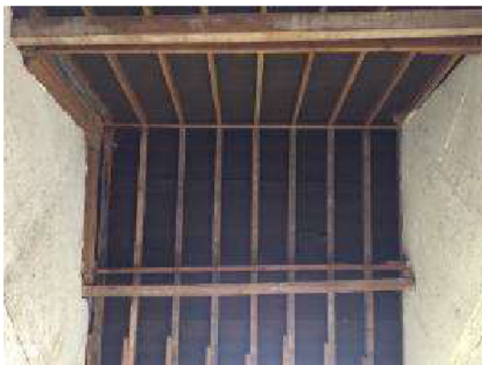
Plates 15 and 16: Barn 1 – Central room (left) and east room (right) showing traditional bituminous felt lining (left – central room) and more recently installed plastic roof lining (right – east room).
