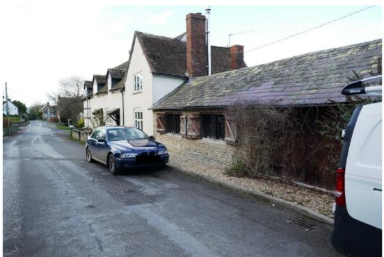
The complex is a vernacular building utilising locally sourced materials with oak framing, wattle and daub infil panels and argillaceous siltstone random rubble masonry set below a plain clay tile roof.
