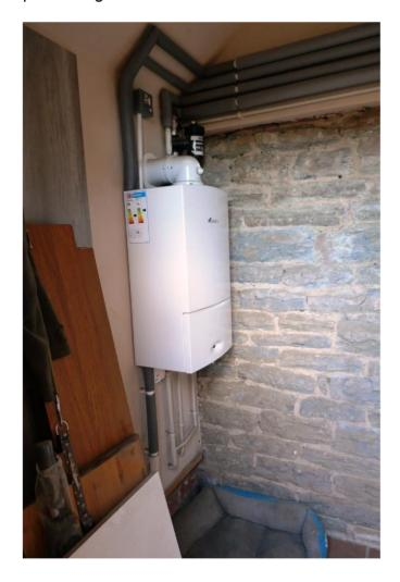
Throughout installation and connection to the existing heating system, pipes have been routed around any decorative or structural element avoiding damage to items of significance.
