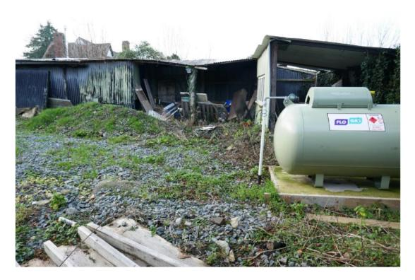
The interconnecting pipework has been laid below ground and is only brought to the surface where drainage pipes preclude further concealement. This location is at the rear of the property close to the new porch and does not compromise any sensitive aesthetic composition. The short runs of pipework to the boiler and onwards under the eaves to the kitchen have been colour coordinated to the host building and constitute a discreet additive change which can be removed without damage to the
