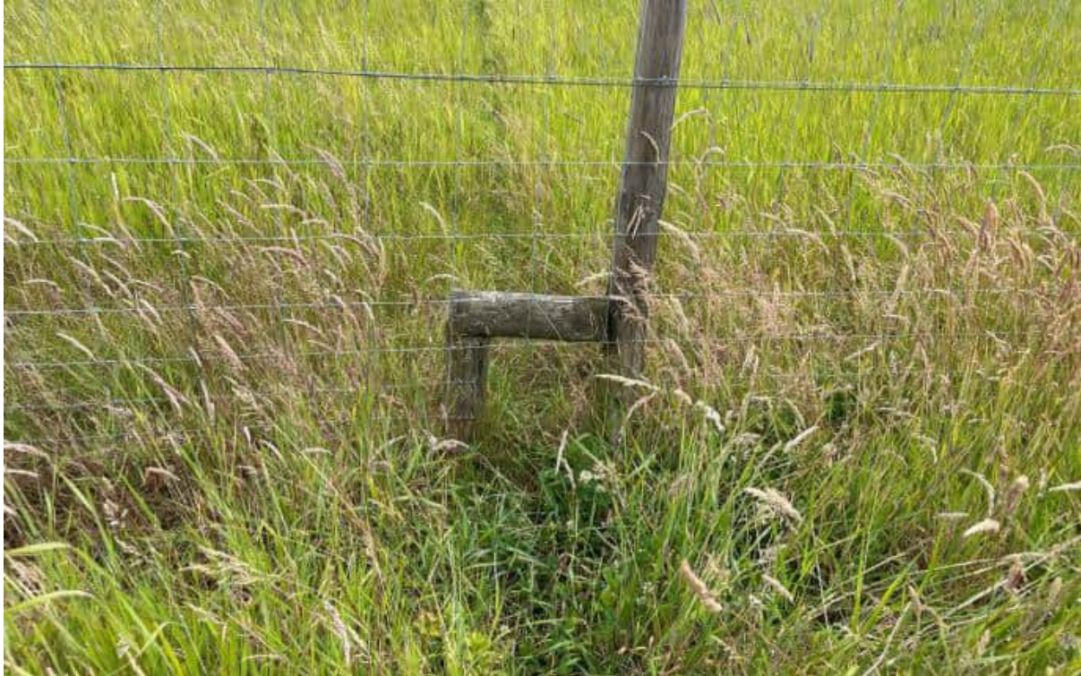
Plate 15: Example of an open mammal gate in the perimeter fencing of a solar farm
