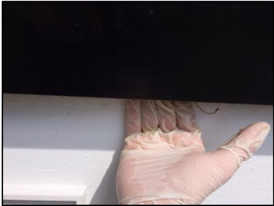
Plate 3: view of gap behind fascia board.
