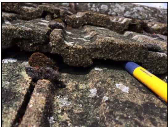
Plate 5: example of crevice along line of lifted tiles on dormer.
