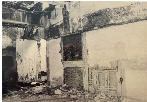
Figure 12: Substantial timber beams with timber framing and wattle and daub infill.
