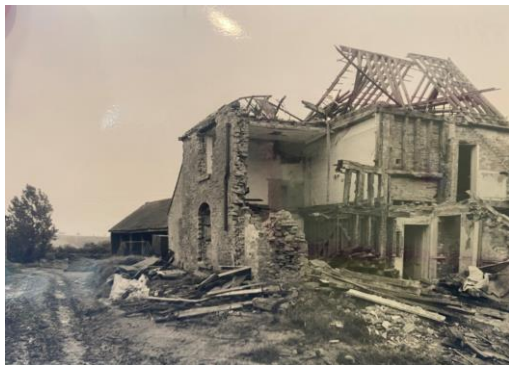
Figure 11: Grendon Court demolition showing timber framing.
