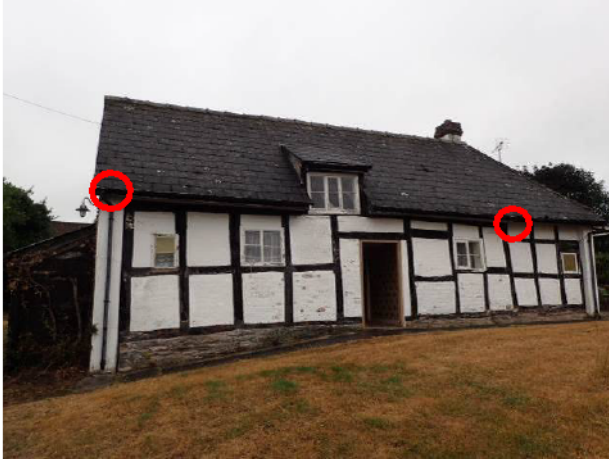
Photo 3: North-eastern elevation and gaps behind weatherboard and bargeboard
