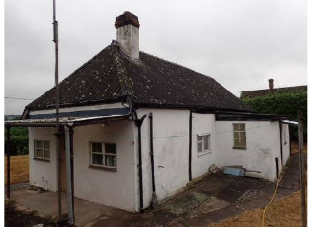
Photo 4: Eastern elevation and missing ridge caps
