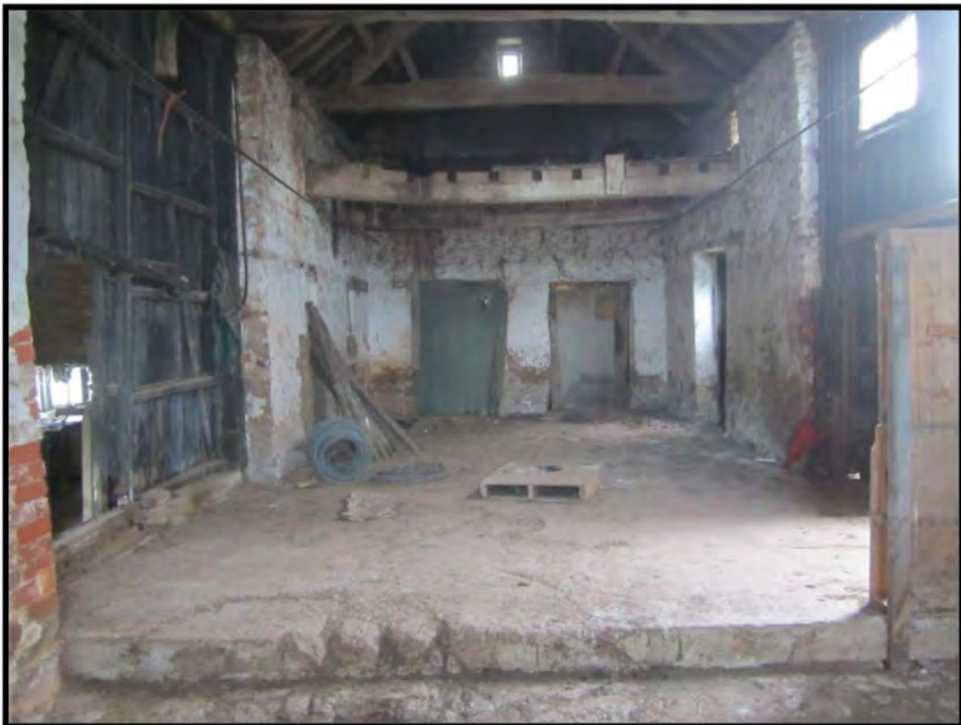
Photograph P12 : showing internal north side
