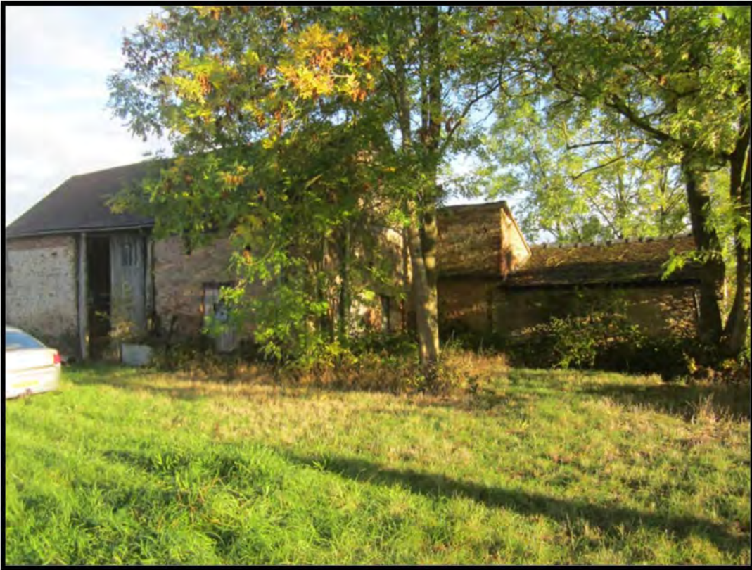
Photograph P1 : showing northwest elevation of barn
