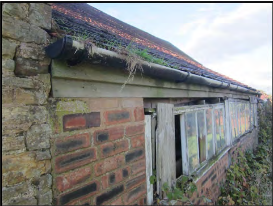
Photograph P2 : showing clay-tiled roof and plastic guttering
