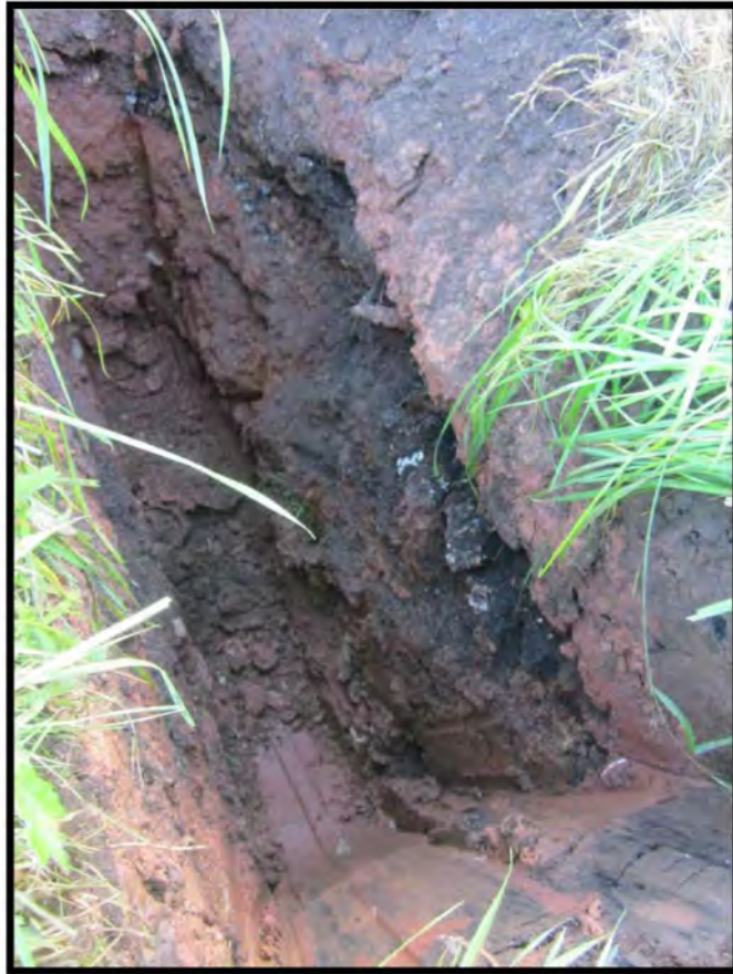
Photograph P9 : showing TP3 showing backfilled pond
