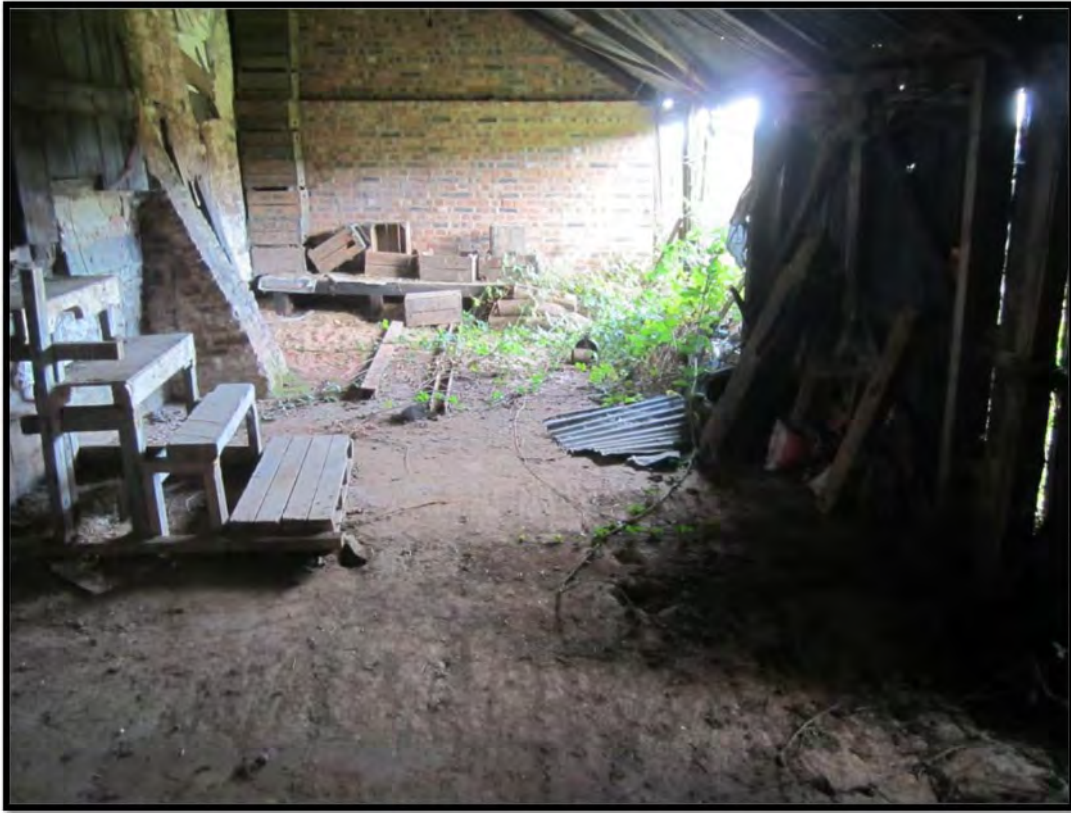
Photograph P11 : showing internal south side
