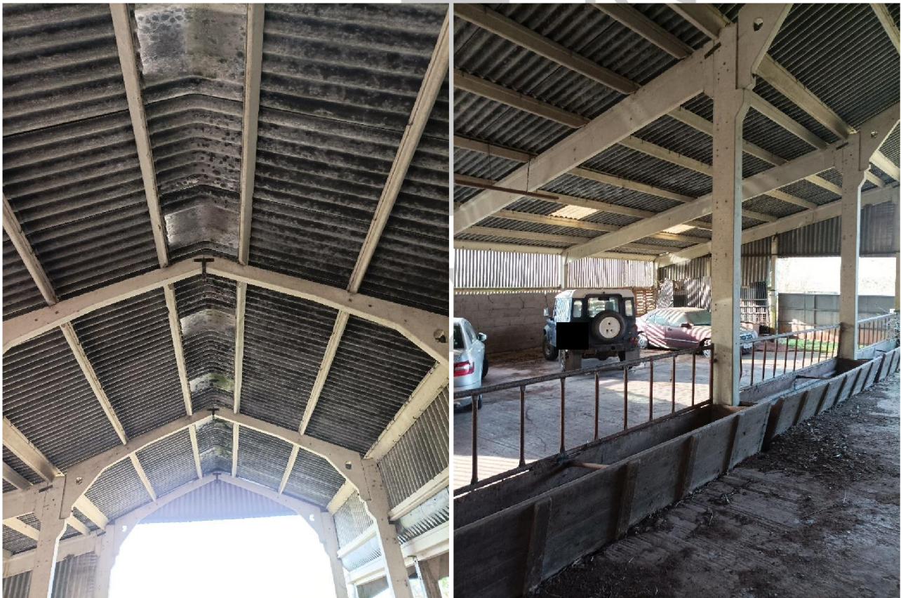
Photo 1: (Left) Portal frame Photo 2 (Right) Lean to
