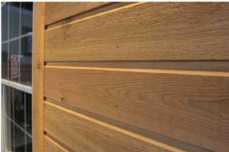
Horizontal cedar shiplap boards.
