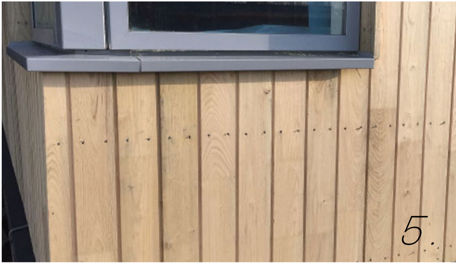
5. ALUMINIUM AND TIMBER CLADDING photo credit: timber2U
