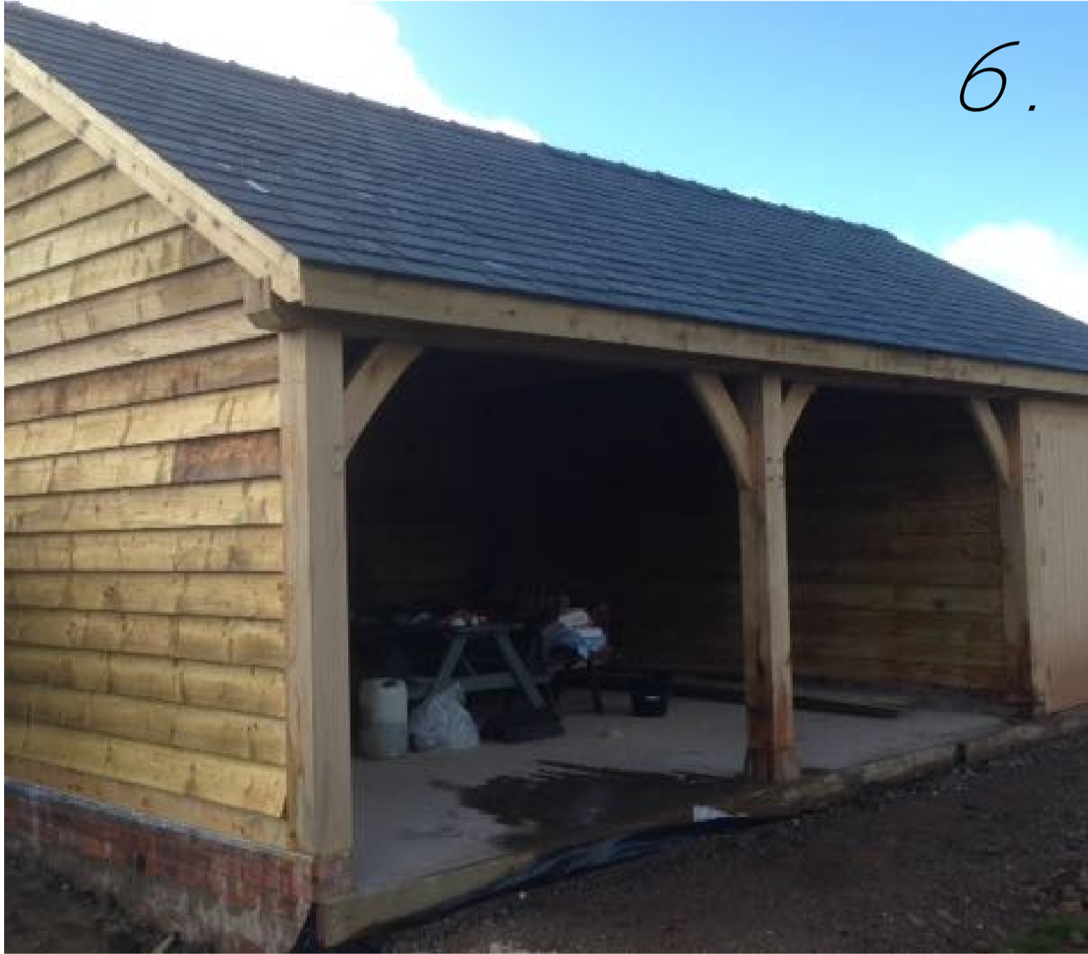
6. OAK FRAME AND WELSH SLATE photo credit: Wye Oak Timber Framing
