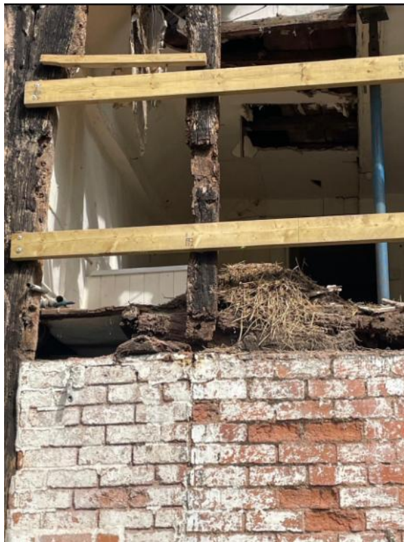
Rear gable end during stabilization works.
