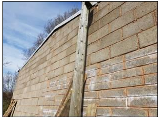
Photo 4 – Gaps at south roof-wall junction verge
