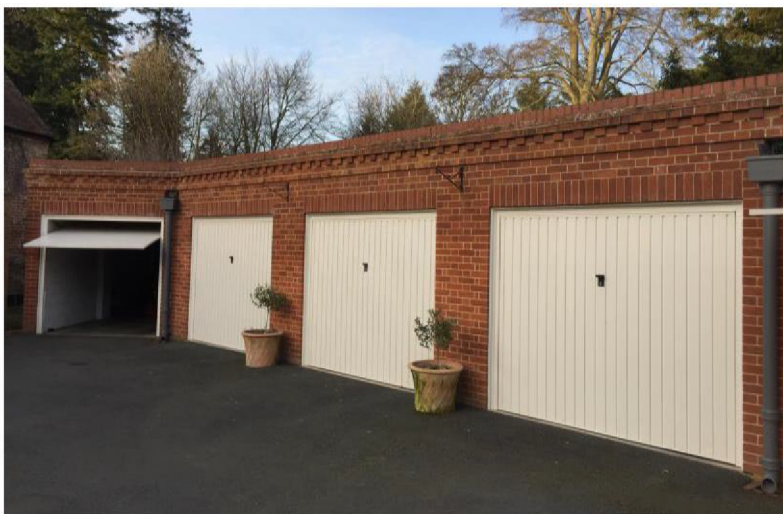
Steel up and over doors to the garage.
