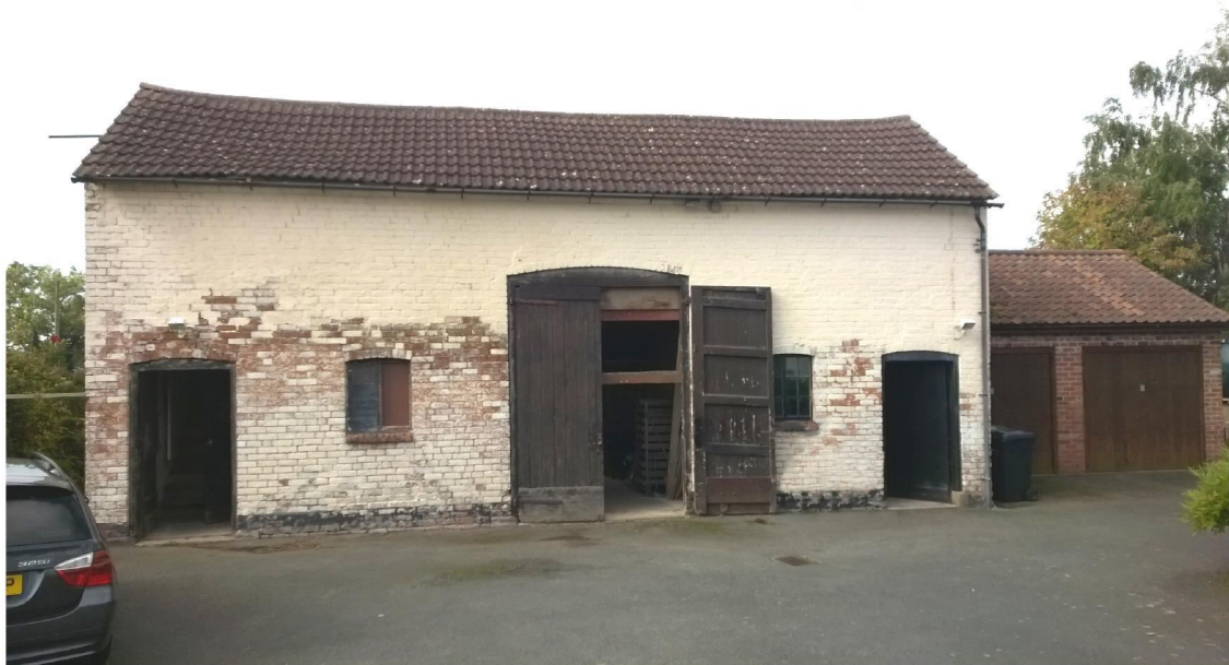
Existing east elevation – note severe roof deflection due to inappropriate replacement roof covering.
