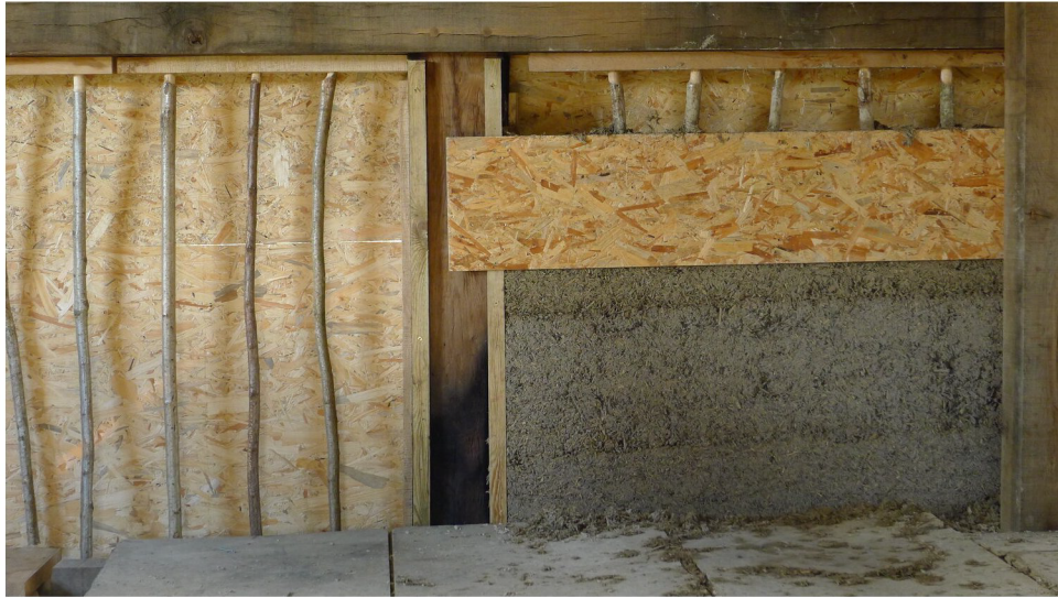
Example image: Showing hazel stakes, and shuttering during the infill process - and right - Finished panel
