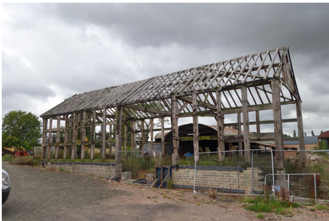
Plate 3: View SE showing N elevation of threshing barn showing intact upper portions of box-framing with reconstructed plinth and sill plates beneath
