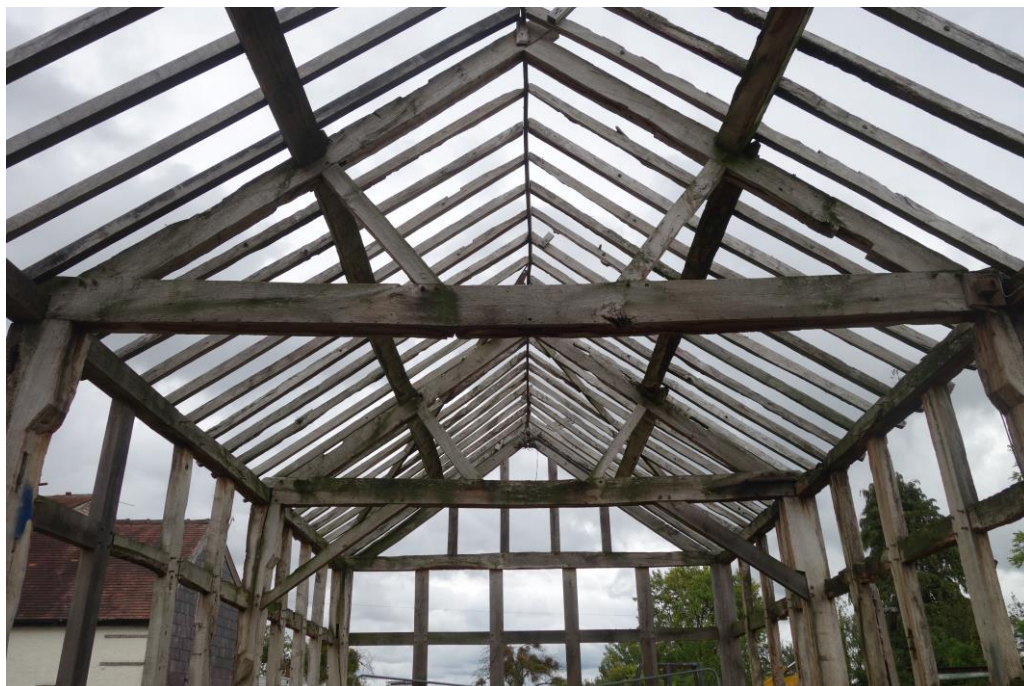
Plate 11: View looking E showing detail of roof trusses in easternmost two bays of threshing barn with carpenter's marks
