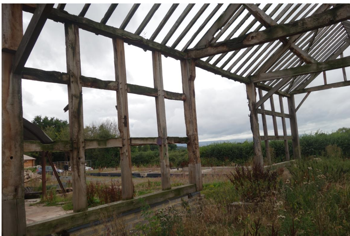
Plate 8: Oblique view looking SW showing detail of framing in S elevation of threshing barn with stave holes for wattled panels and slots for internal partitions
