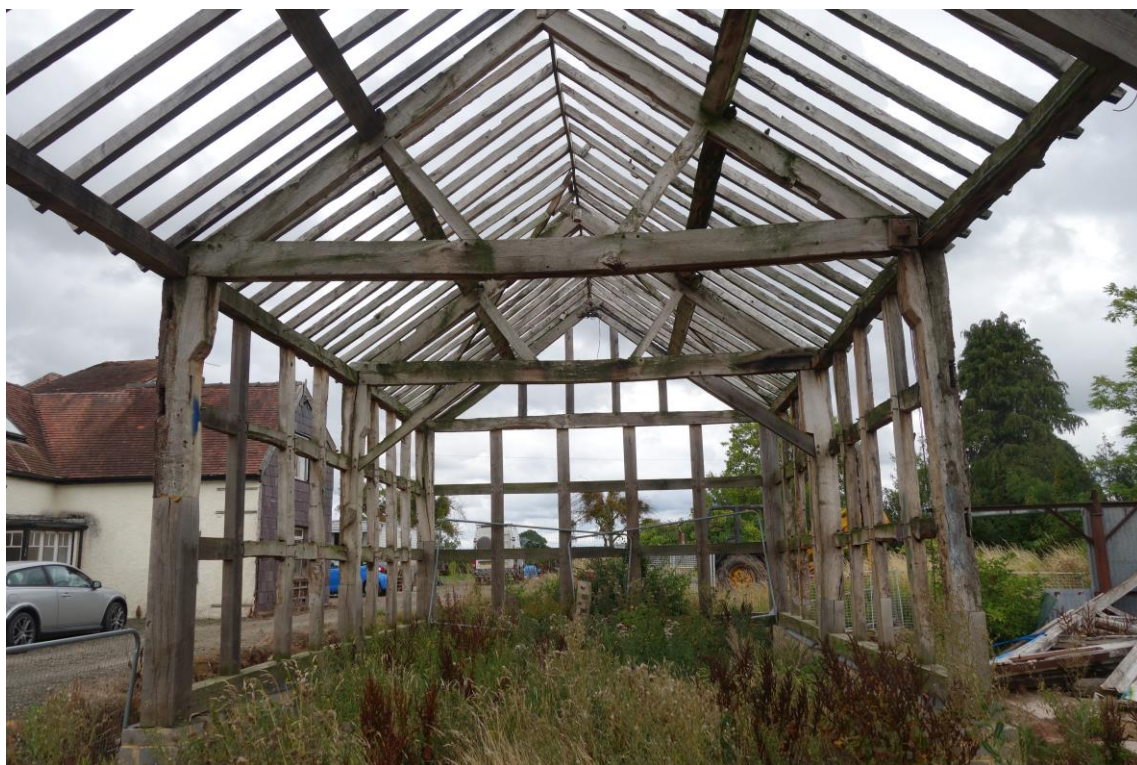
Plate 9: View looking E showing interior of central and easternmost two bays of threshing barn with open-truss roof structure and trenched purlins
