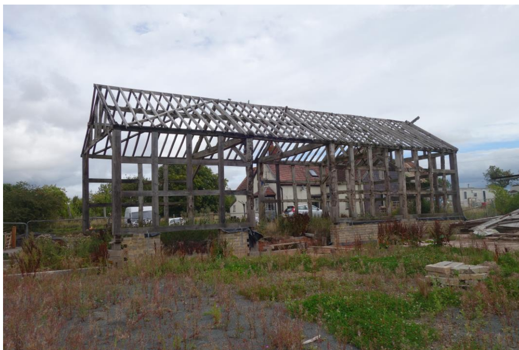
Plate 1: View looking NE towards threshing barn showing reconstructed plinth and sill plates, with farmhouse to rear
