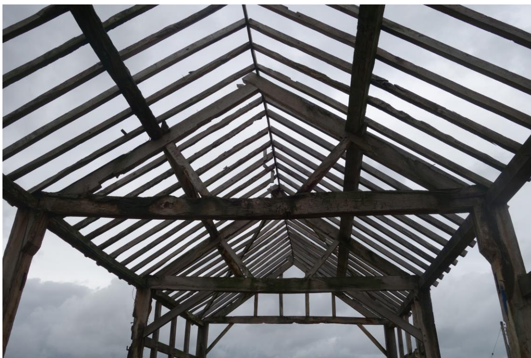
Plate 10: View looking W showing detail of roof trusses in central and westernmost bays of barn with carpenter's marks
