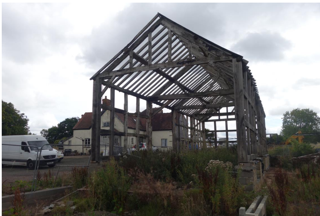
Plate 6: View looking NE showing extant framing in apex of W gable end of the threshing barn comprising four vertical struts, with the remaining framing removed
