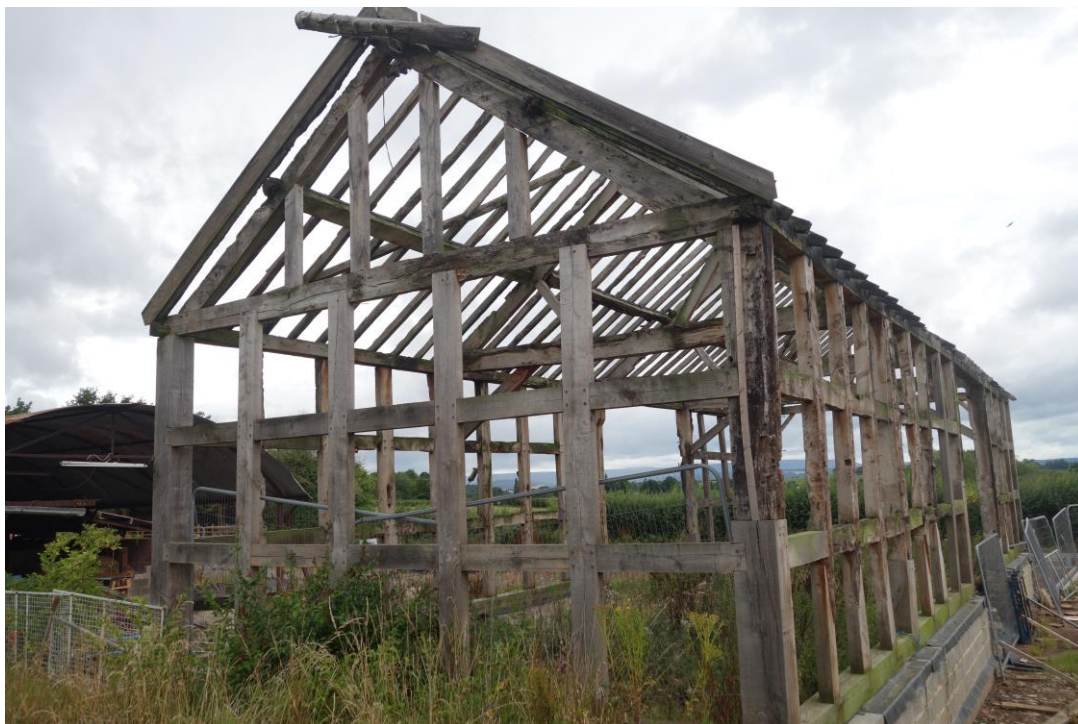
Plate 5: View SW showing E gable end of threshing barn with reconstructed box framing and original framing in the apex of the gable consisting of four vertical struts
