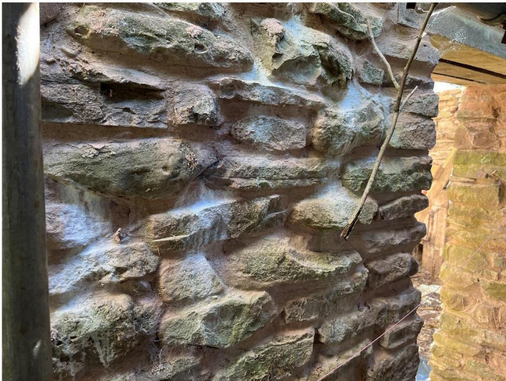
Plate 2. Stonework has been recently repointed.
