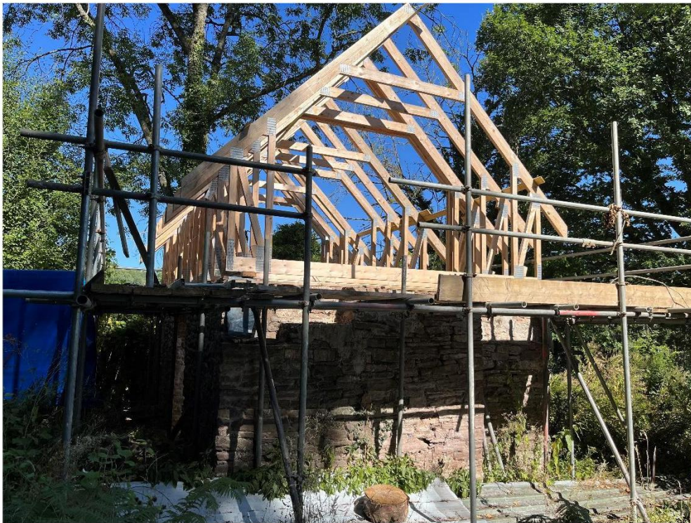
Plate 1. The derelict stone cottage with new roofing timbers.
