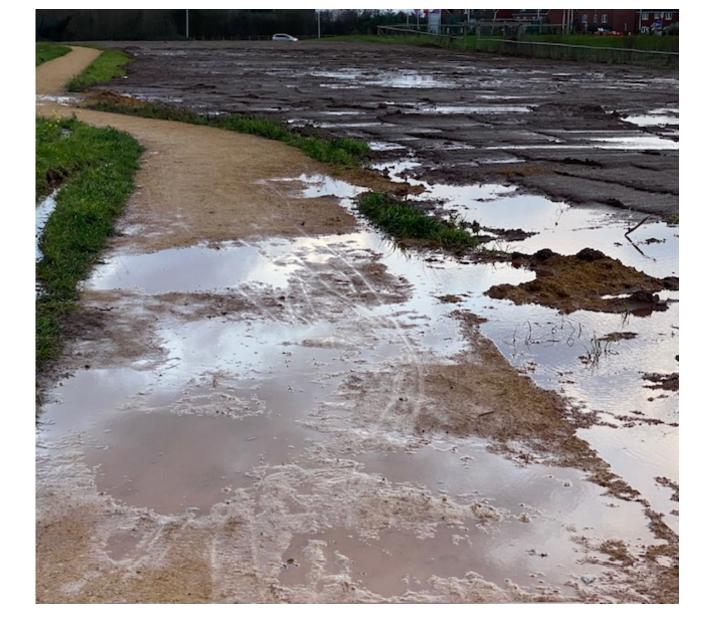
7. Natural drainage of the site is poor partly due to the clay subsoil moved onto the site by the developers. There is insufficient planning for rainwater drainage from the large area of building in this application, particularly with consideration of the continued flooding in Ross.
