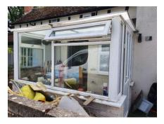
Reinstated porch works have started (floor dimensions 2100cm x 2400cm) Block work base on raised concrete pad with oak framing and pitch roof to bring the porch more in keeping with the original property.
