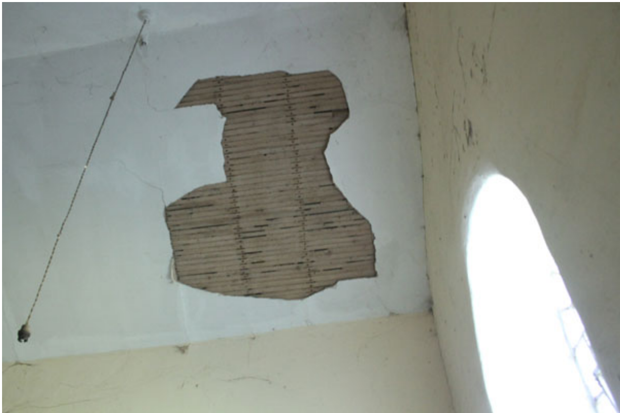
Plate 7: shows the ceiling of the main internal room, including exposed wooden laths
