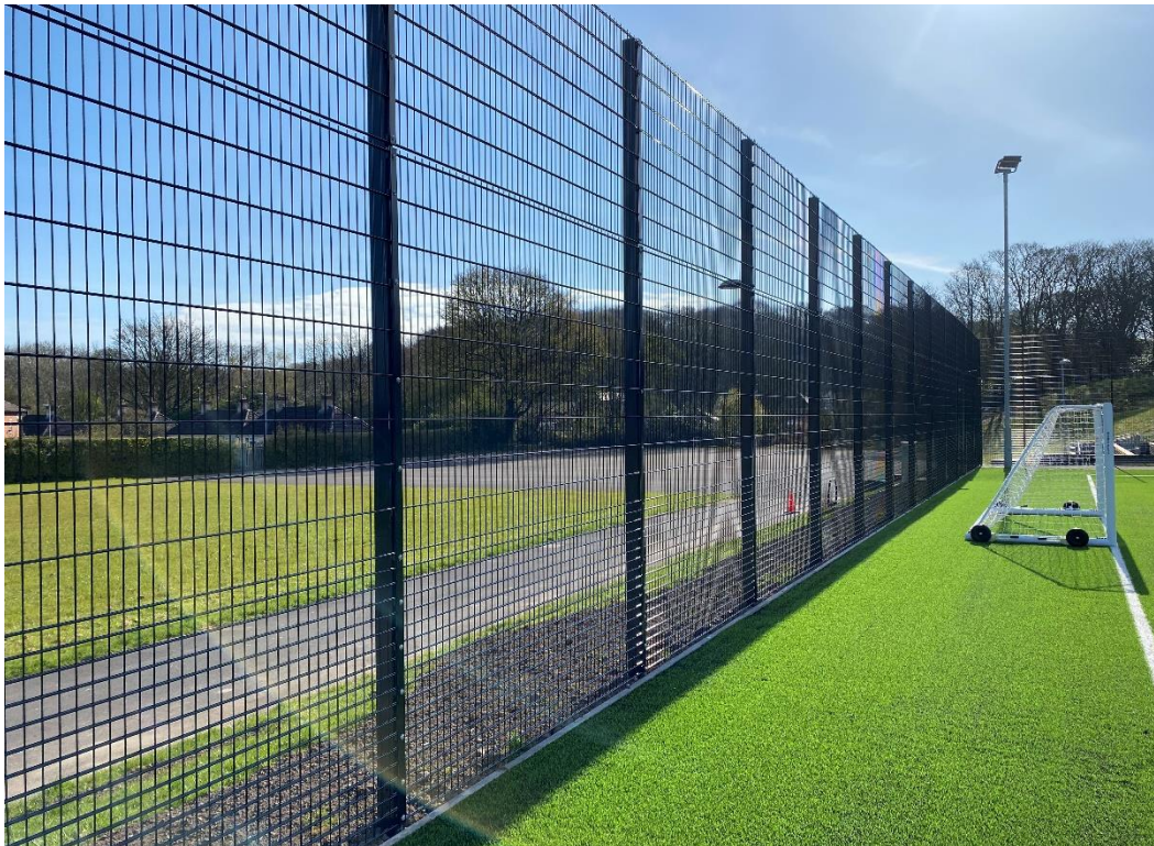
4.5m high open mesh type fence, powder coated black RAL 9005
